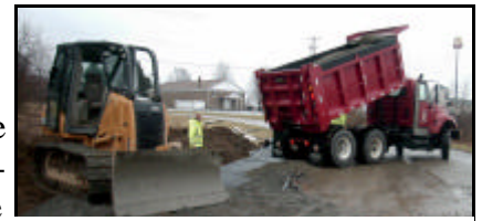
Todd Reynolds, Lawrence Township employee directing Dover Township truck dumping aggregate on emergency roadbed. Click on the Above photo to view slide show.
